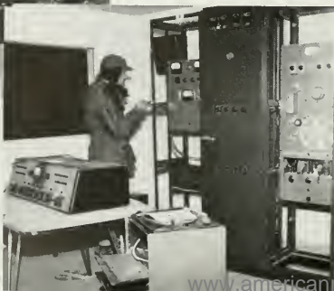
Photos taken before (left) and after (below) atomic blast show that RCA transmitter and associated equipment emerged with only minor damage.
