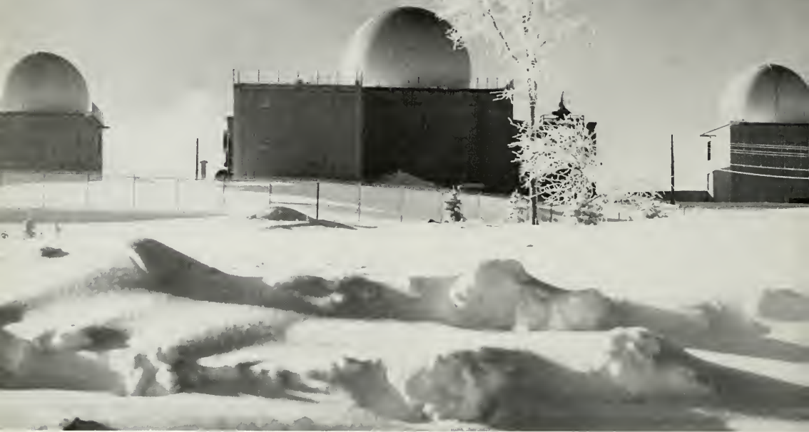
Domes housing electronic equipment stand against winter sky at an RCAF radar station.
